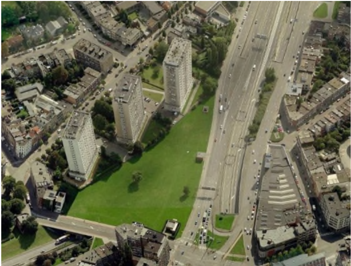
Figure 2 Aerial view of the high-rise apartment building site that is to be refurbished (image from Google Maps)
